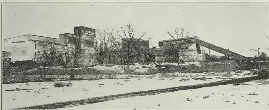
Fig. 30. Plant of National Silica Company, Oregon, Illinois. On the left is the building housing the screening and pulverizing machinery, and just behind the tree in the center of the picture is the circular draining bin. The other buildings house the power plant and washing and drying equipment. (Photograph by courtesy of National Silica Company.)
